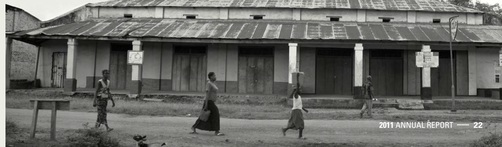
Rehabilitation Center site Dungu, DRC
